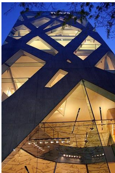
Arh. Toyo Ito, TOD'S Omotesando , Tokyo (2004) Sursa: http://structurehub.com
